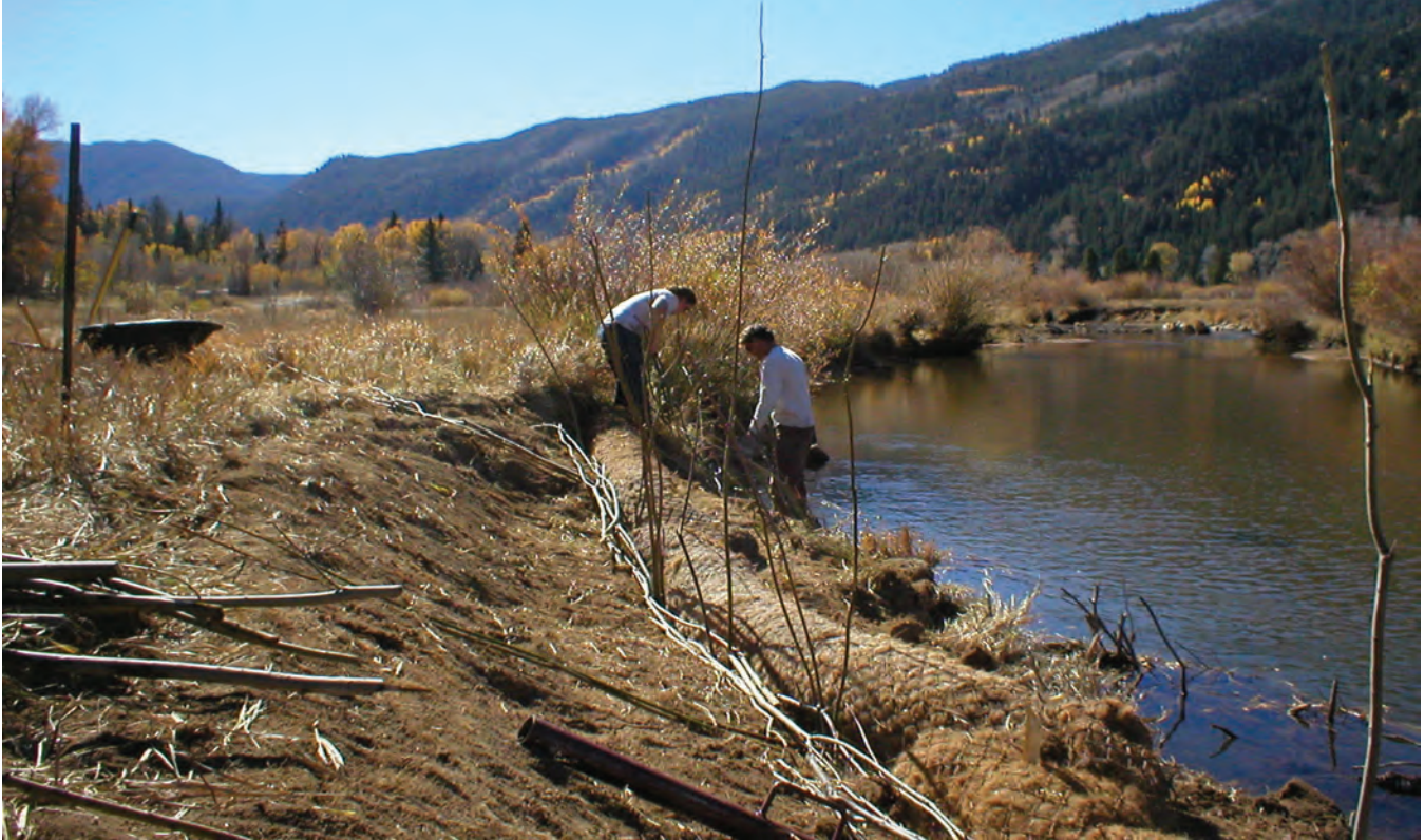
Above and below: Previous efforts at steambank restoration at North Star.
