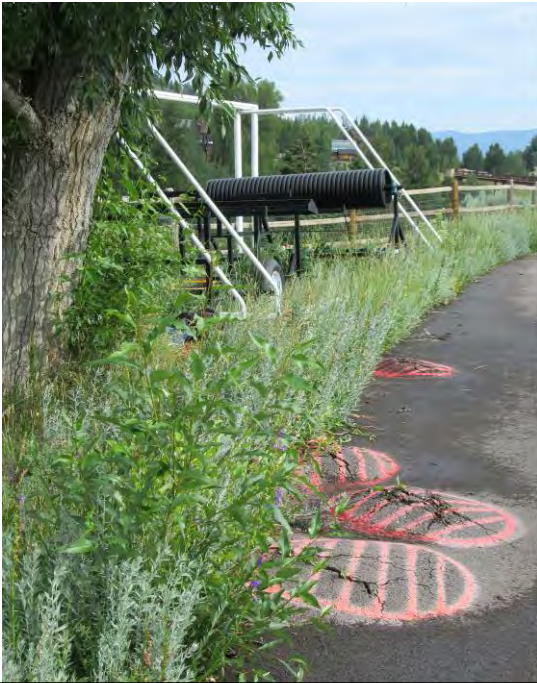
Figure 14. Narrowleaf cottonwood's root are affecting the sidewalk by lifting it.
